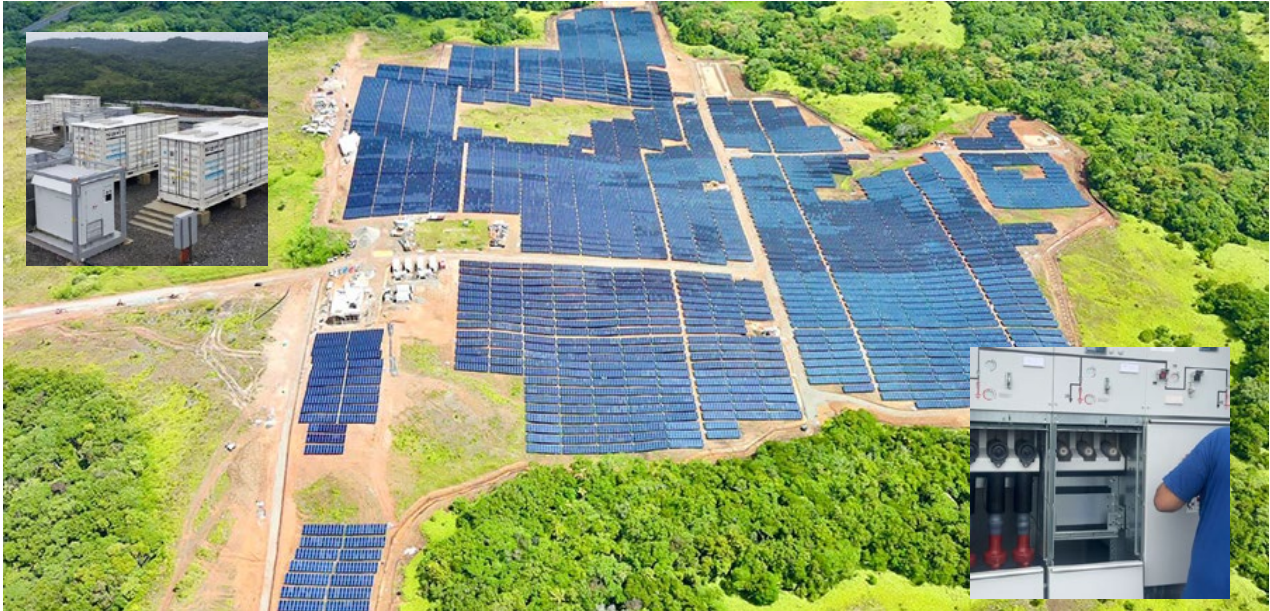
OSINT Source: https://www.sma-sunny.com/en/solar-plus-storage-project-western-pacific-palau/
