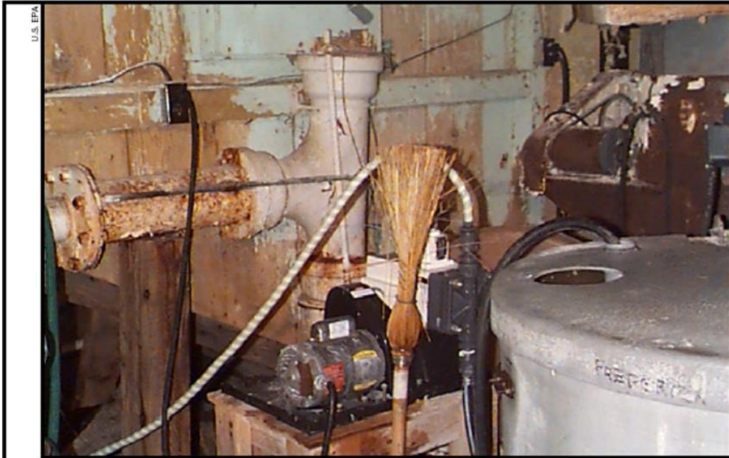
Some water systems employ short-term measures to postpone the expense of replacing and rehabilitating infrastructure. Here a water system uses a broom to prop up a chemical feed line. With a $4.4 million DWSRF loan, a neighboring water system expanded its treatment capacity to serve the community previously served by this deteriorated system.
